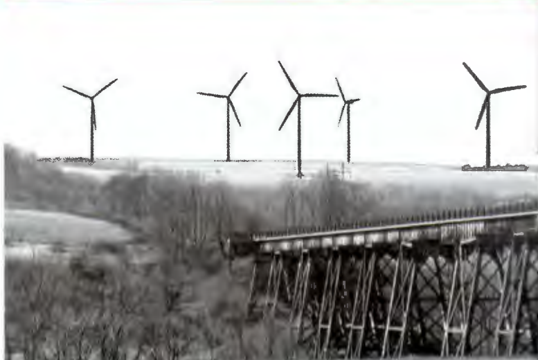
Salisbury Viaduct and Garrett wind farm
