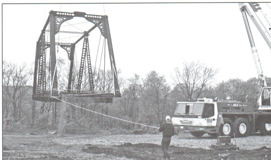
The Bollman Bridge is lifted and swung into an adjacent field.
