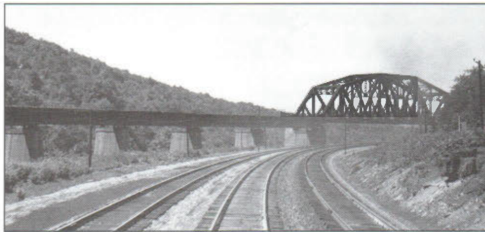
Keystone Viaduct as it looked in 1945 from the rear of a B&O passenger train. The second and third piers from the left and the girders that rest on them will be replaced with a single 240-foot-long girder. (See map, front page)
