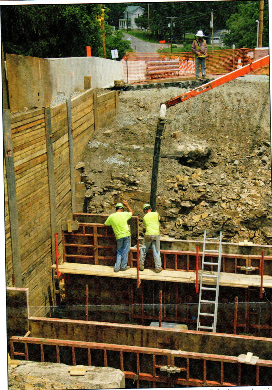
Wing walls are poured where the GAP will pass under Berlin Street in Garrett, eliminating a road crossing.
